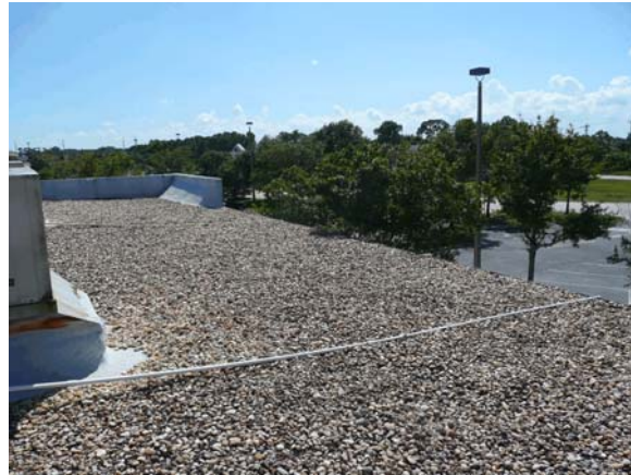
Figure 5: Roof No. 19 with 1.5-inch aggregate and a wrap-around parapet.
