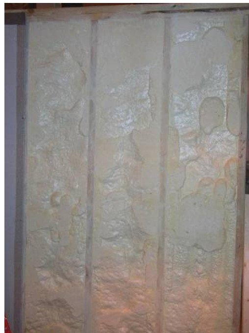
Figure 2. Open-cell spray foam wall
